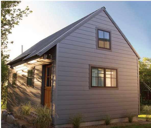
Fiber Cement Board Siding (by Kevin Browne Architecture)
